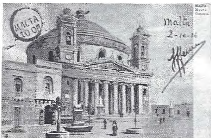
Figure 3: Church in Mosta, Malta
